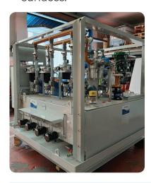
Oil Circulating Systems (Lube Oil Skids) are used to lubricate the Thrust and Guide Bearings on a Hydro Turbine and Generating equipment.
