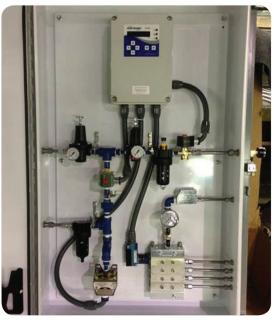
Automatic Grease System in Enclosure
